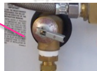
Temperature and Pressure (TP) Valve
